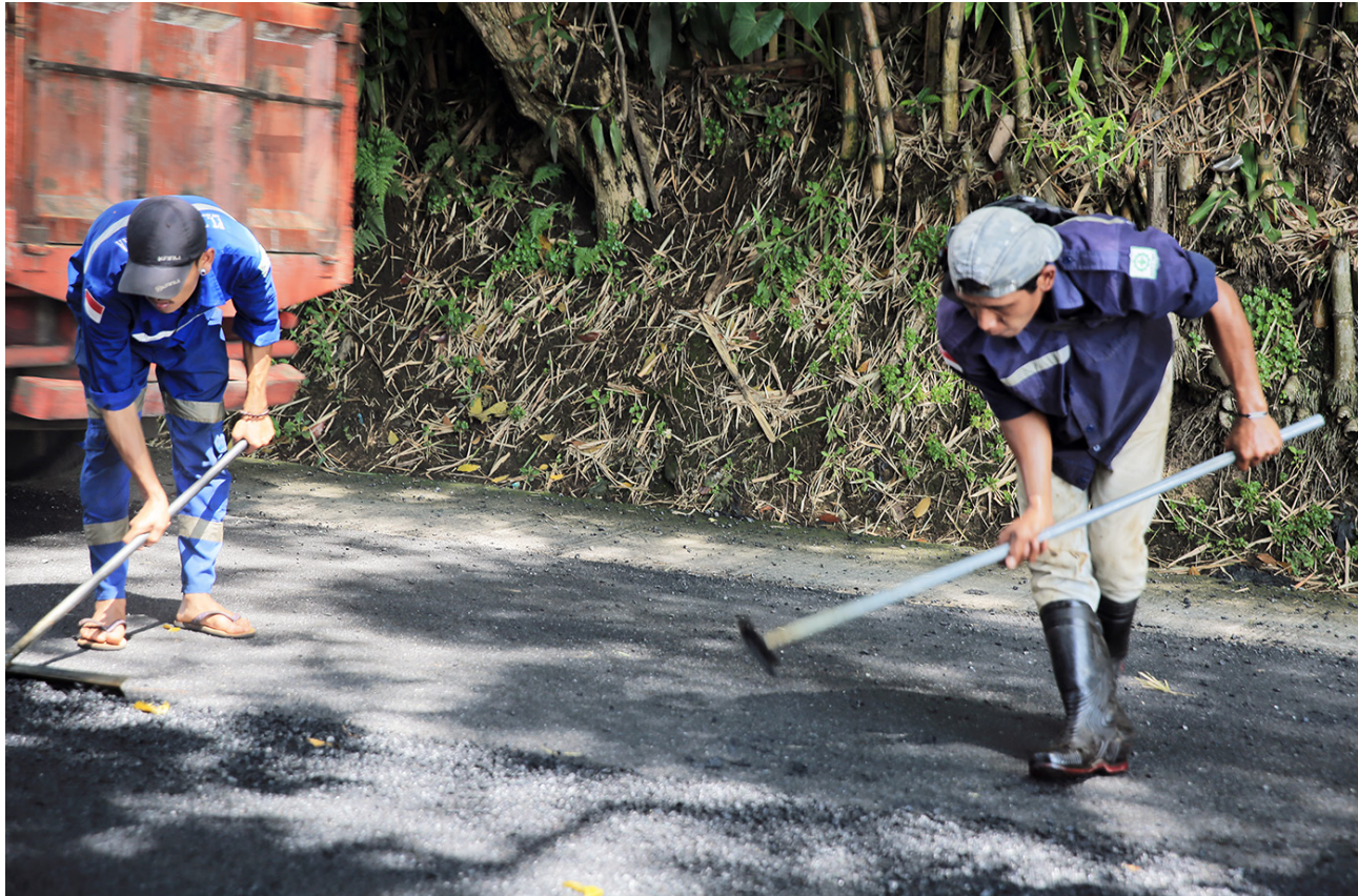
Climate Innovation: Chandra Asri construction workers are laying down plastic asphalt in Garut Regency. Five years ago, the Garut Regency government signed a cooperation agreement with Chandra Asri to build plastic asphalt roads throughout the region.
